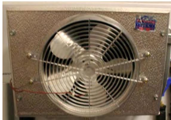
**Figure 2.8 The evaporator unit fan**
